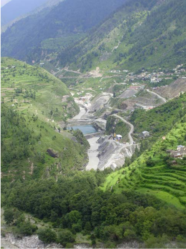
Image 5: Dam at Tapovan Vishnugad under construction. Photo by Kelly Alley [file name: tapovanvishnugaddam2]
