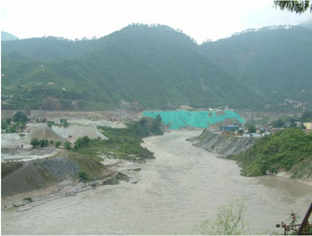
Image 4: Dam at Srinagar, Uttarakhand under construction. Photo by Kelly Alley [file name: Srinagardam1]
