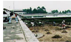
Work is done on a slow sand filter. Courtesy of Dr. N. Nakamoto, Shinshu University.
