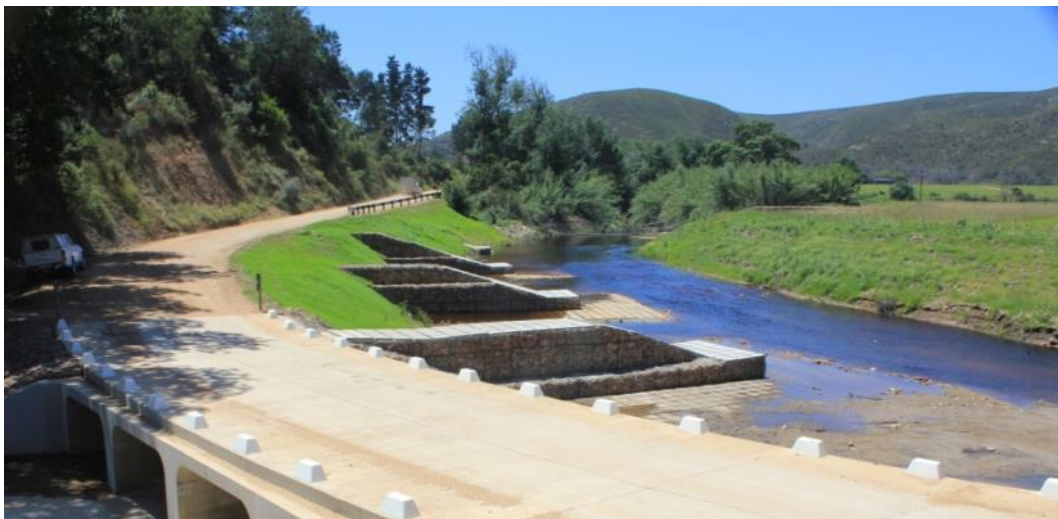
Figure 5 A typical situation where river rehabilitation work on one bank can influence the stability of the opposite bank
