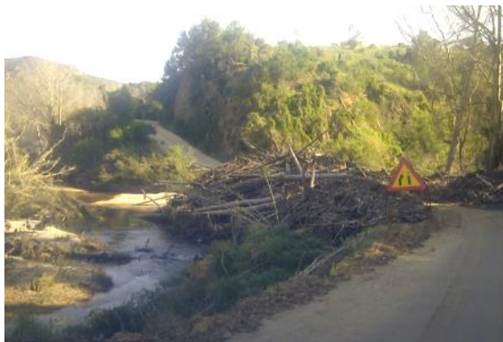
Figure 39 Bottelierskop site 2 : post flood - 2012 (photo R Tyndall, Kantey and Templer)
