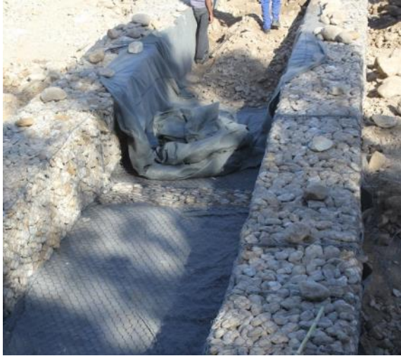
Figure 23 Preparing envelope for cellular construction - note the mesh below the geotextile envelope
