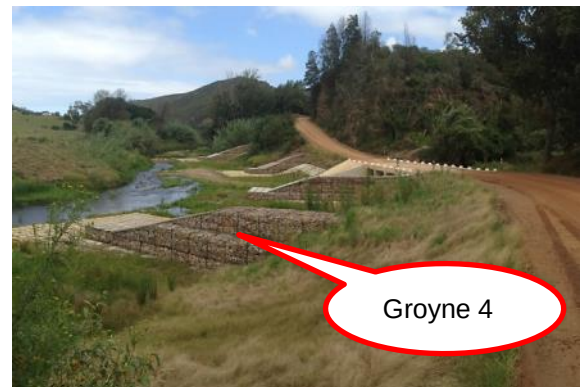
Figure 40 Bottelierskop site 2 : post construction - 2015
