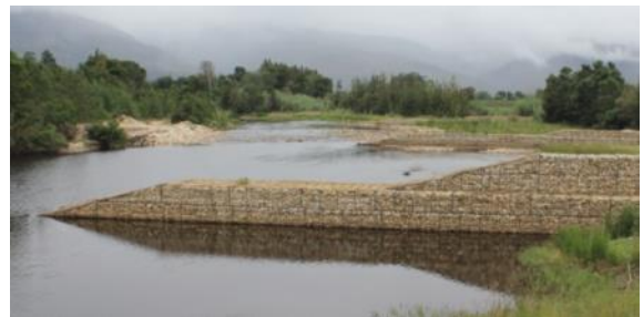
Figure 22 A more recent Western Cape groyne showing the sloped tip which greatly reduces scour.
