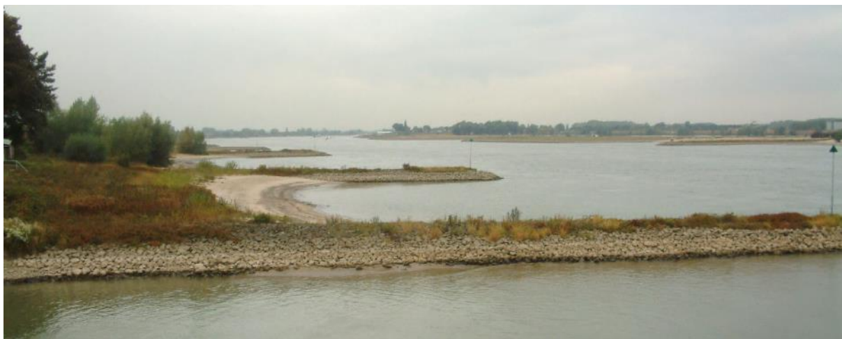
Figure 8 Groynes on the Waal River at Zaltbommel (Netherlands)
