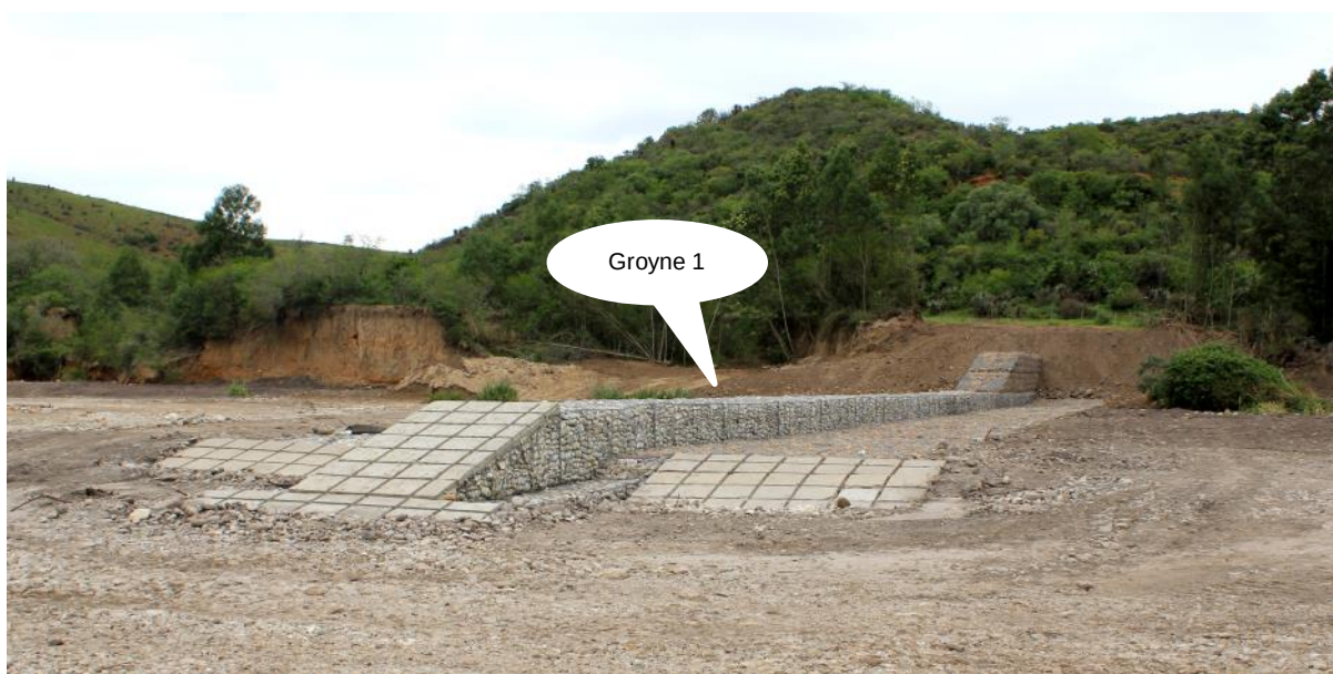
Figure 44 View of most upstream groyne (groyne 1) showing its length relative to its height – its function is mainly to locate the fast flowing channel away from the river bank
