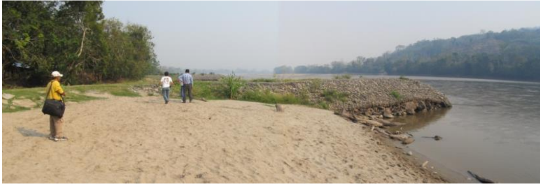
Figure 4 Erosion control groyne on bank of Upper Amazon at Campanilla, Peru. The river is too wide for the structure to influence the opposite bank
