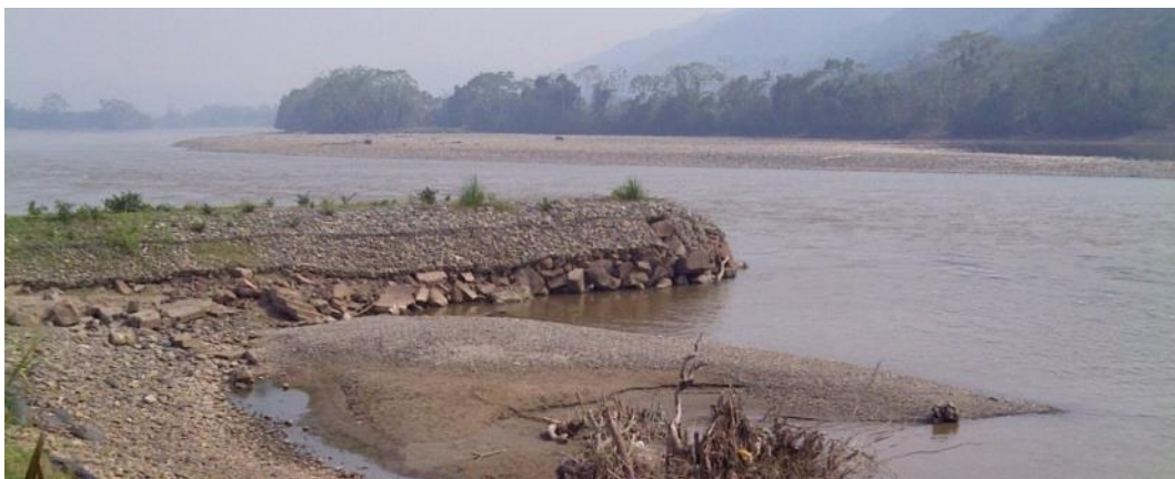
Figure 12 Groyne on the Huallaga River at Campanilla (Peru)
