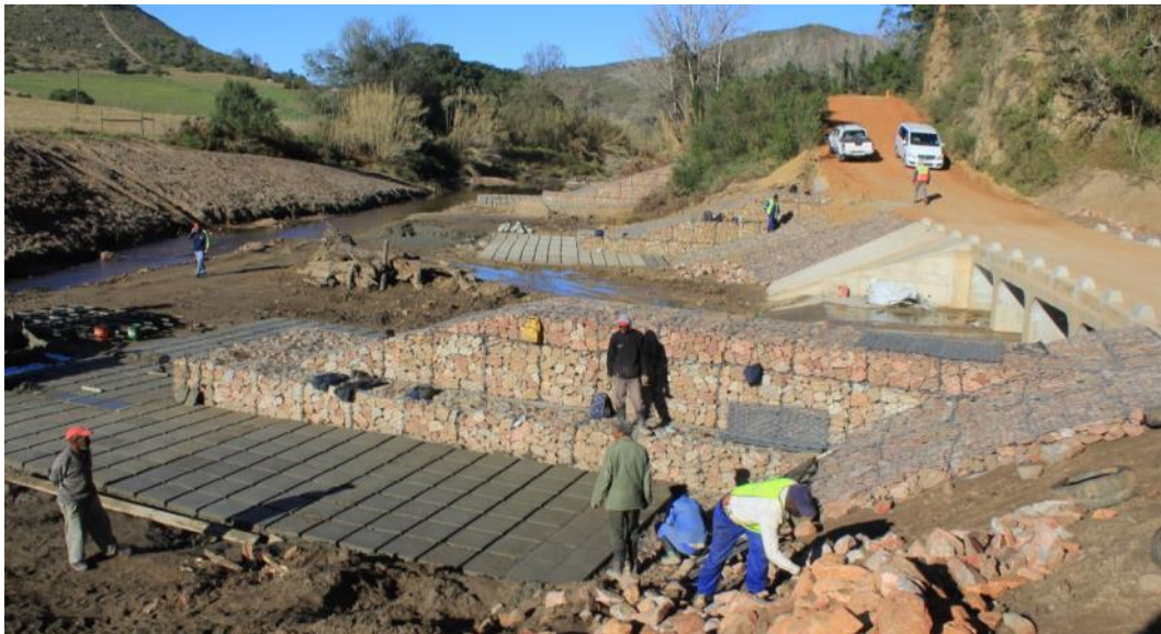
Figure 25 The provision of concrete abrasion pads to gabion mattresses around tip of groyne
