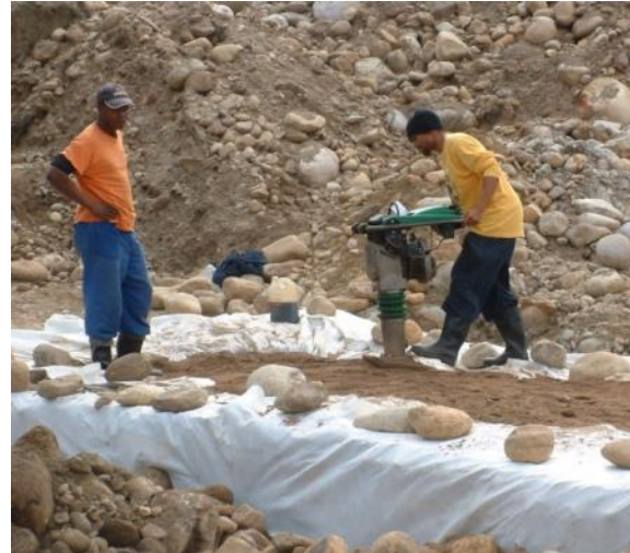
Figure 24 Compacting the granular fill in the envelope before closing and sealing
