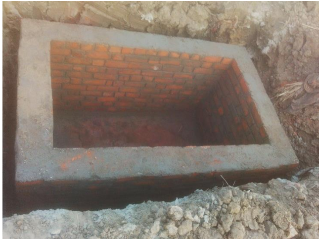
Clearford One™ ClearDigest™ Smart Digester™ tanks Under Construction
